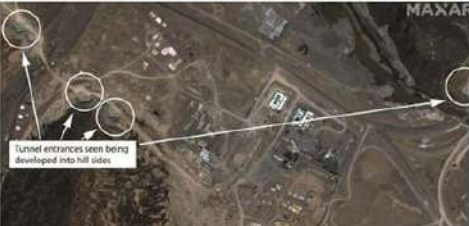
Tunnel entrances seen being developed into hill sides
